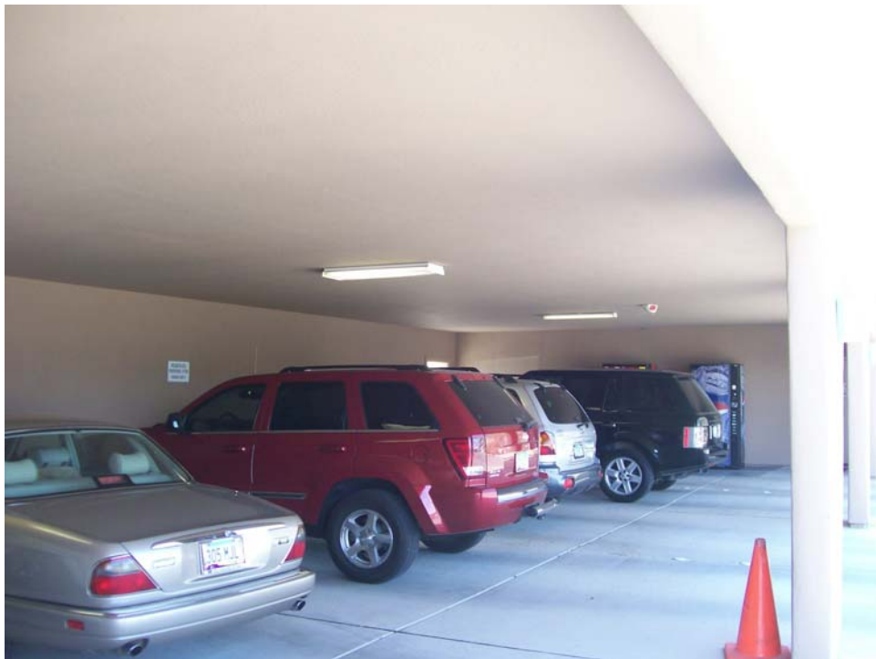
Subject – parking garage
