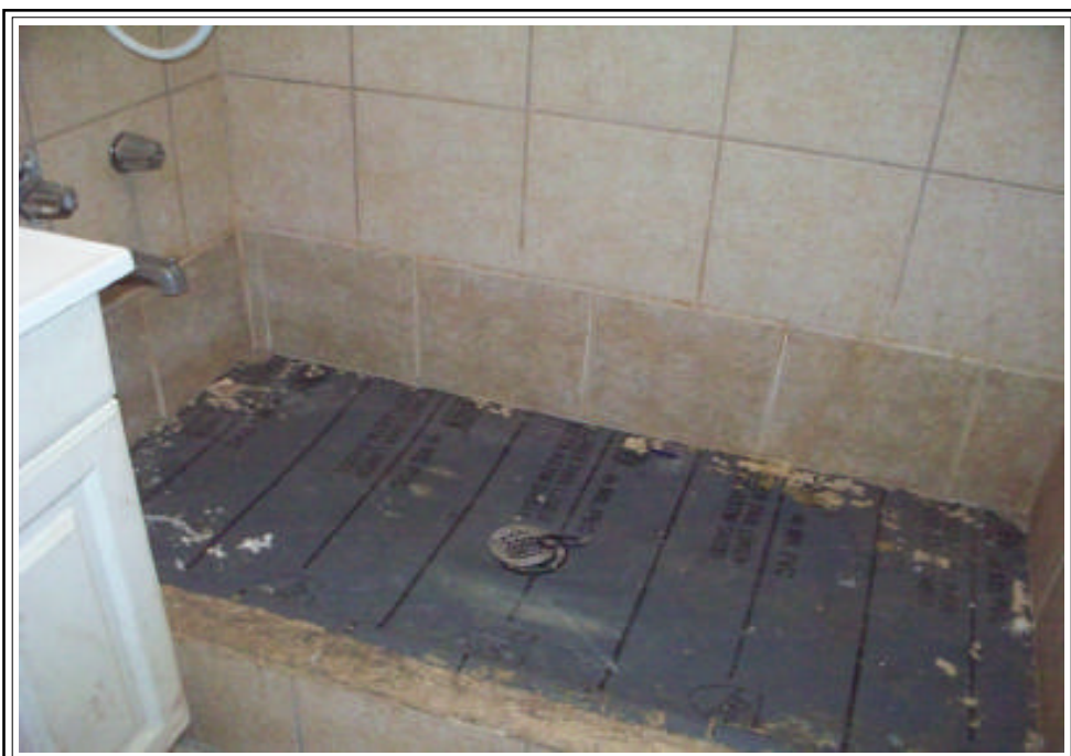
Unfinished shower in Bathroom
