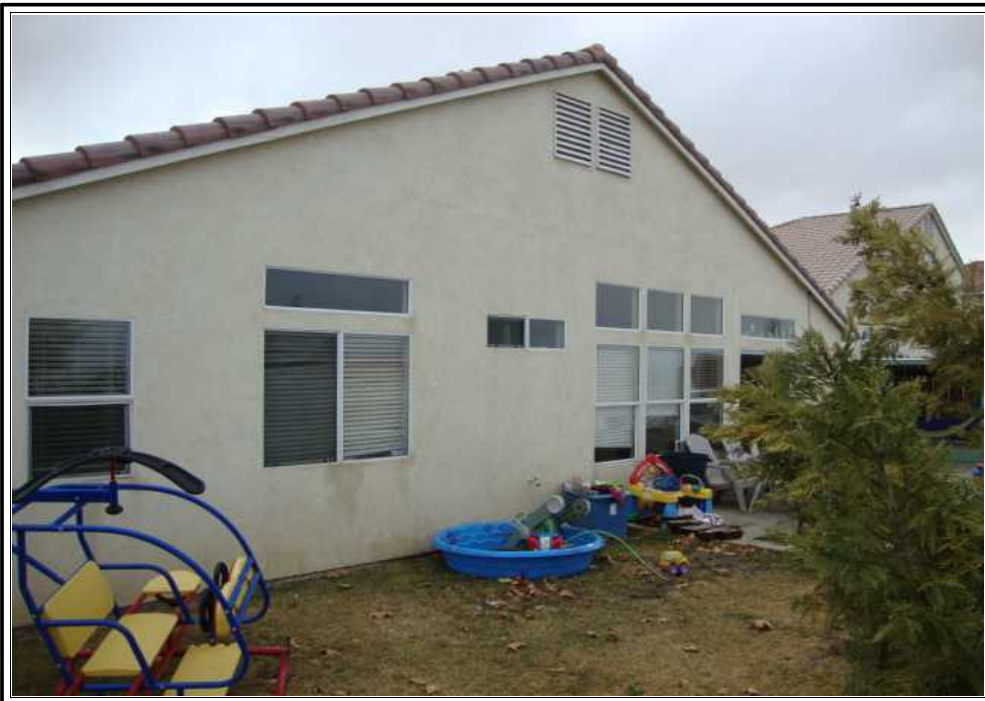
REAR OF SUBJECT PROPERTY
