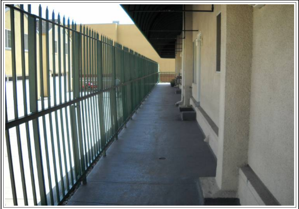
Walkway to front entrance.
