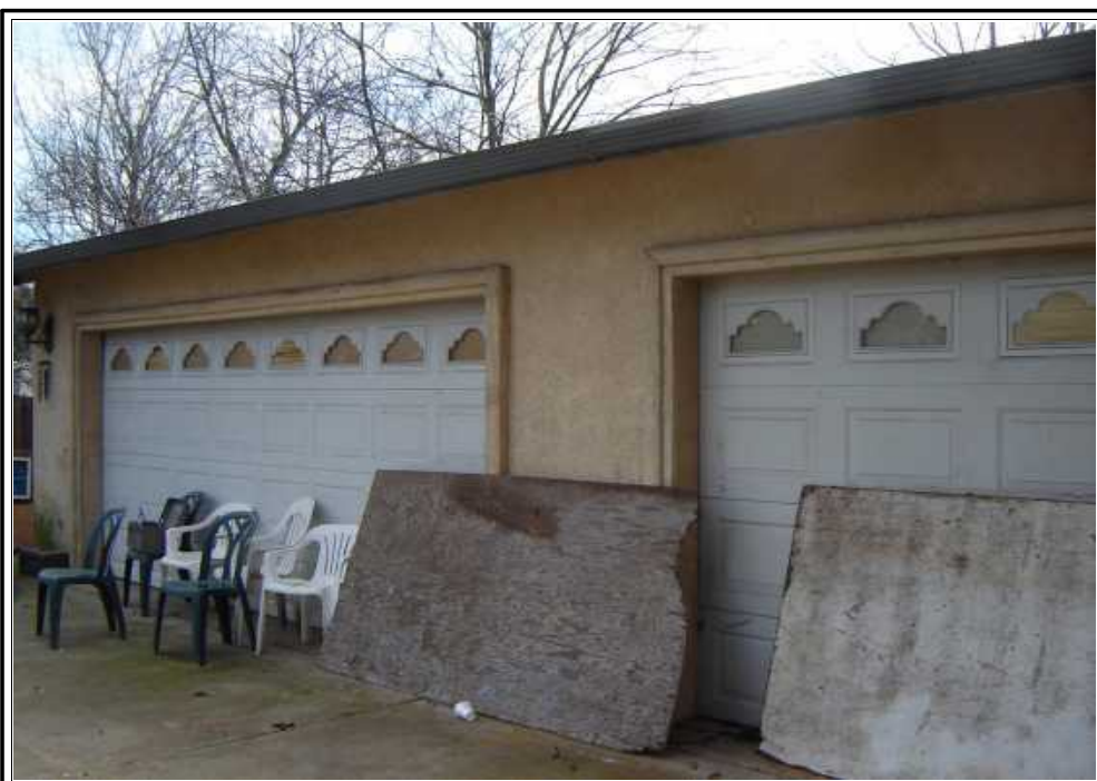
Detached three car garage -Not accessible from the street-
