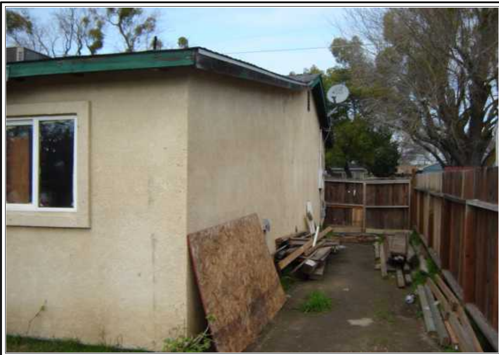
Left side view of subject -This is the only access to garage-
