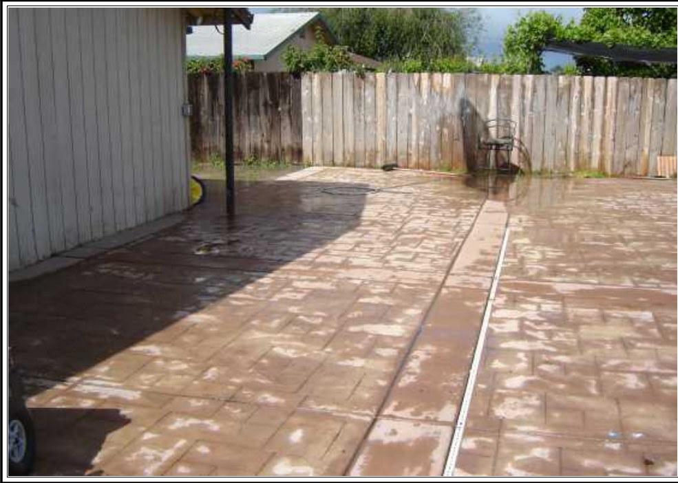
Stamped concrete patio
