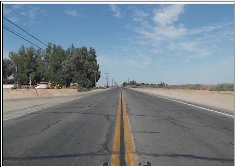
Hwy. 98 looking east
