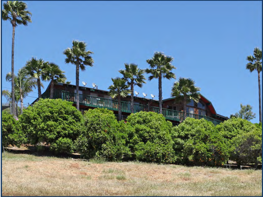
DATA NO. 3 1178 EVERGREEN LANE, VISTA
