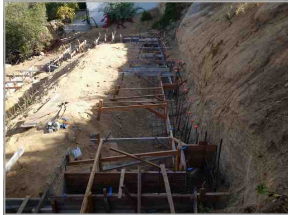
Upper Foundation Forms
