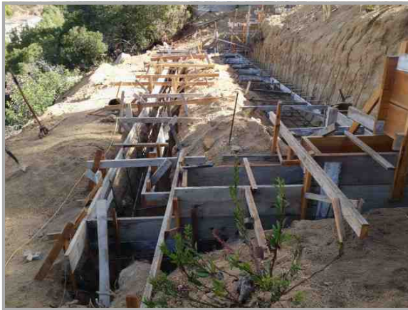
Lower Foundation Forms
